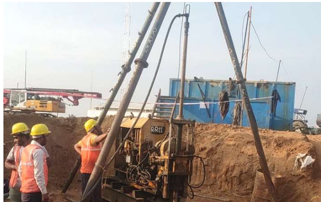
Fig. 7. Pile Coring in Progress
