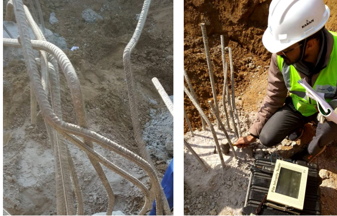
Fig. 5. Pile integrity tests in progress
